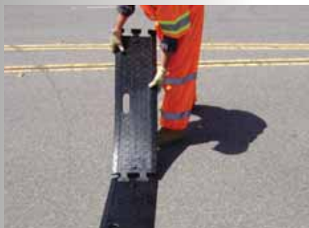
Jigsaw connection for secure and simple deployment
